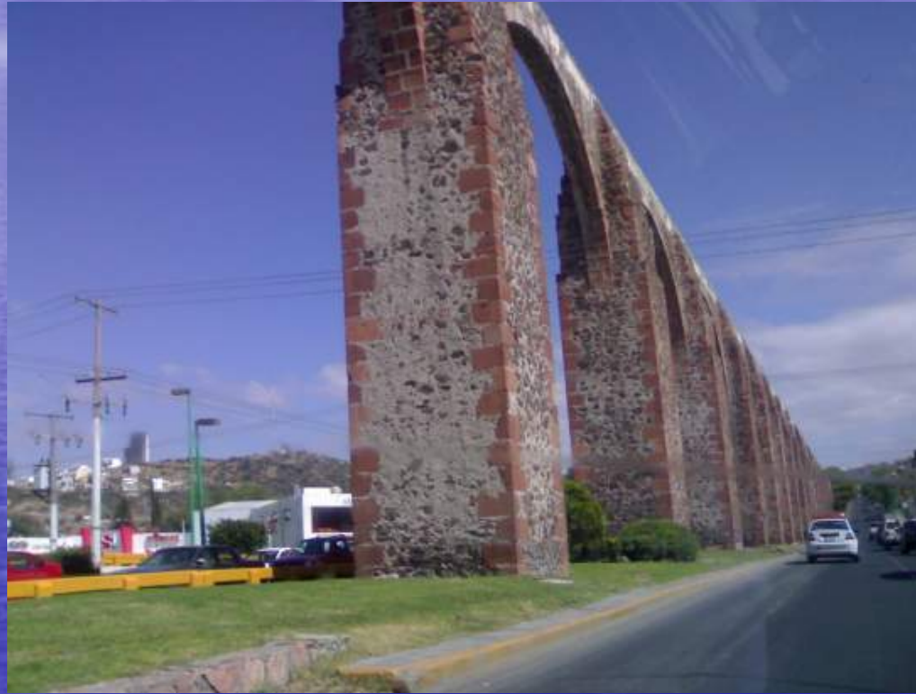
The historic city of Queretaro The aqueduct – built to carry water to the city
