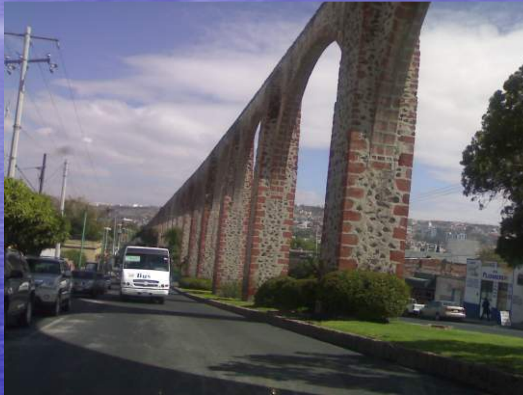
The historic city of Queretaro The aqueduct – built to carry water to the city
